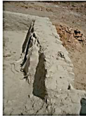
The successful use of the geo membrane, whose life is almost 100 years, this process is successfully used on the steps area, where it has been, membrane and then mud plaster is applied.
